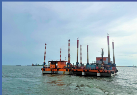
Soil investigation works for Tuas Port Phase 3 using jack-up barge
