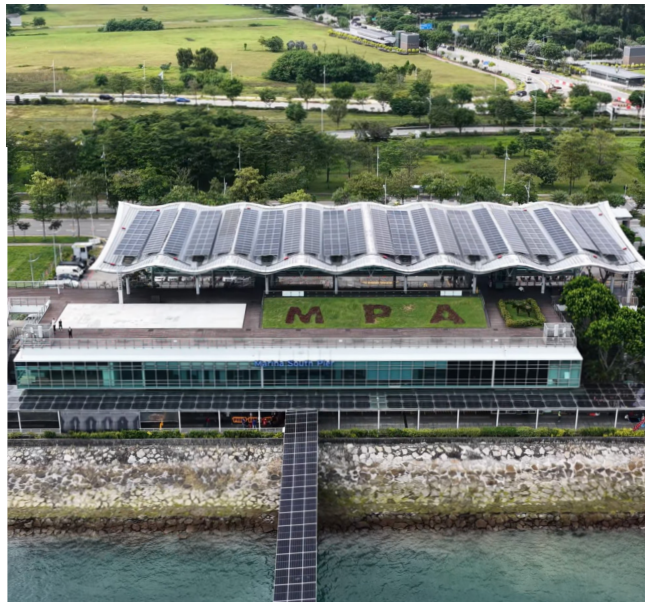
Solar Panels at Marina South Pier
