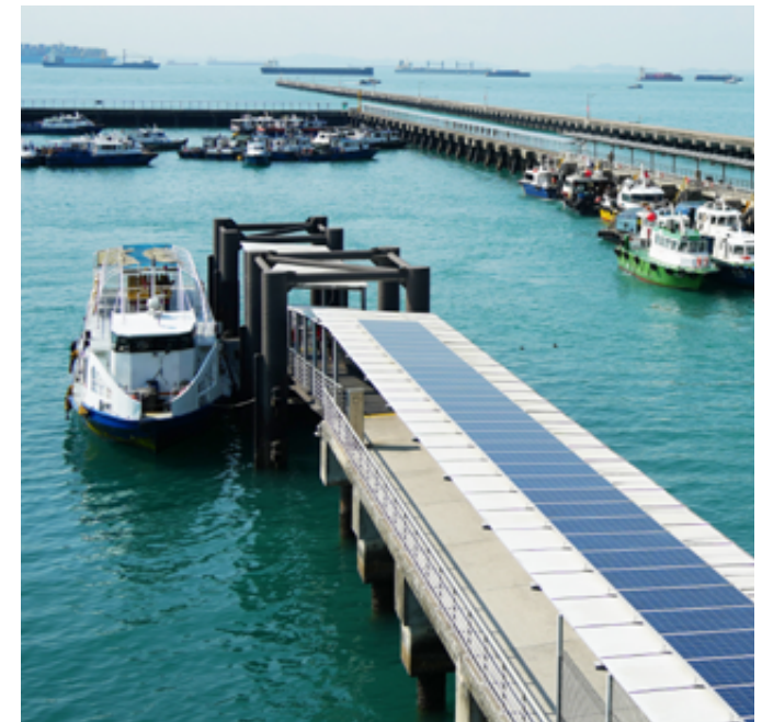
Solar photovoltaic panels at Marina South Pier
