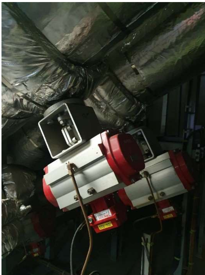
Exhaust gas damper actuators
