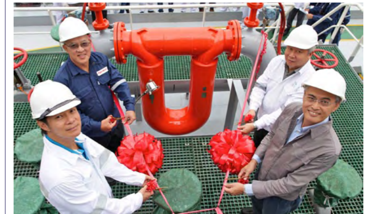
Launch of the first mass flow metering system for commercial delivery in Singapore in July 2012.
