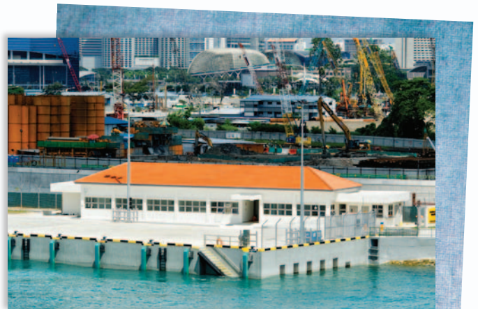
Marina South Wharves provides better berthing and support facilities for lighters.
