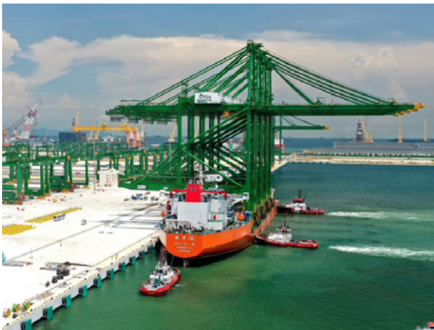
Quay Cranes being delivered and installed at Tuas in the earlier part of 2021
