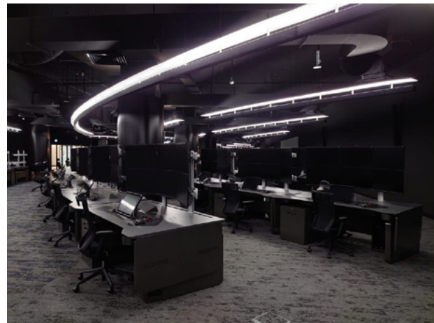
Control centre for Tuas Terminal ready for operations
