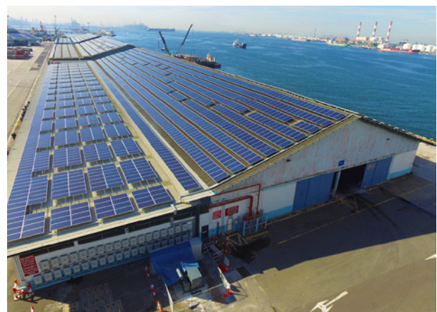
Solar panels at Jurong Port
