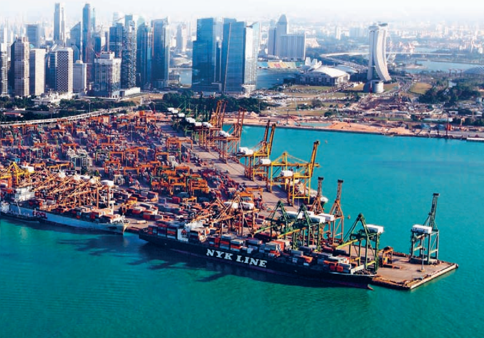
ABOVE: PSA has been a leader in applying technology in container terminals, pioneering PORTNET, CITOS and remote crane operations.
