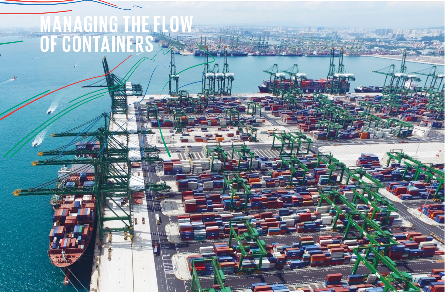
ABOVE Both remote-controlled and automated crane systems are in use at Pasir Panjang Terminal.
