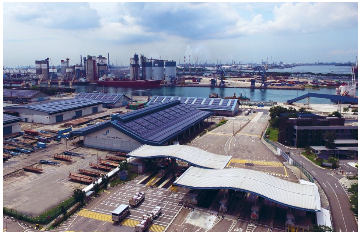
RIGHT An aerial view of Jurong Port. FACING PAGE Training at Jurong Port Academy covers different aspects of port operations, including specialised courses on operating port equipment such as the sideloader.
