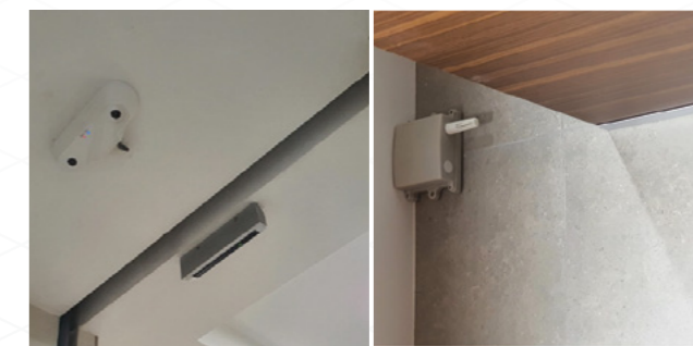
Ammonia and human traffic sensors installed in the washrooms of MPA's mTower office
