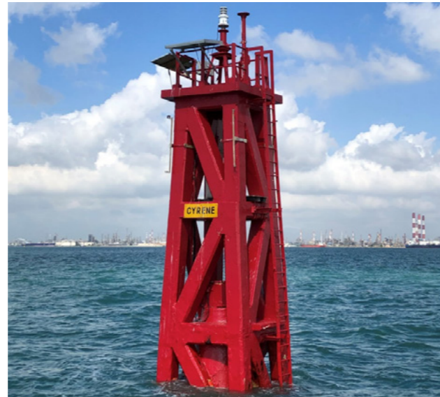
A dual intensity LED lantern installed on Cyrene Beacon
