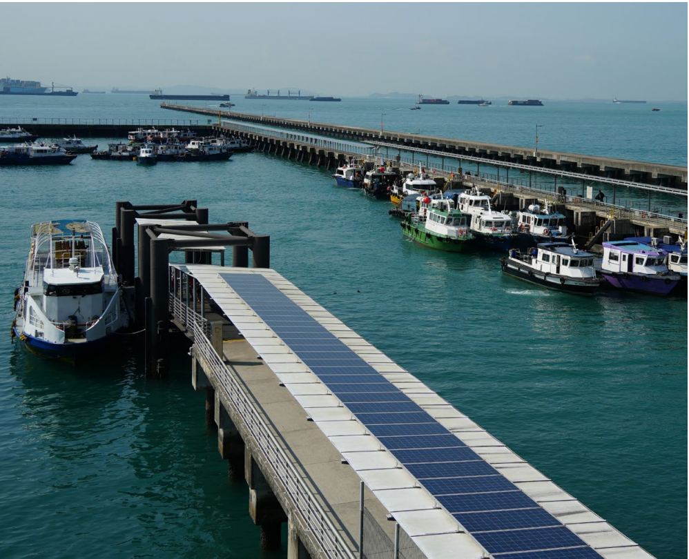
Solar photovoltaic panels at Marina South Pier.
