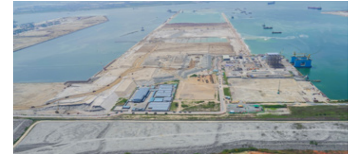
Developments at Tuas Port Phase Two.
