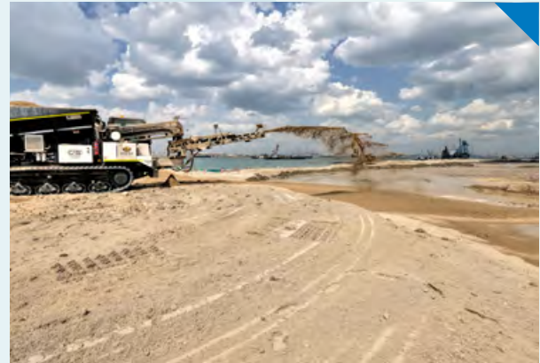
↗ Reclamation work using Conveyor Application System (CAS)
